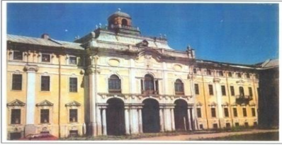
Figure 22: View from the Southern Facade of Konstantinovsky (19)
